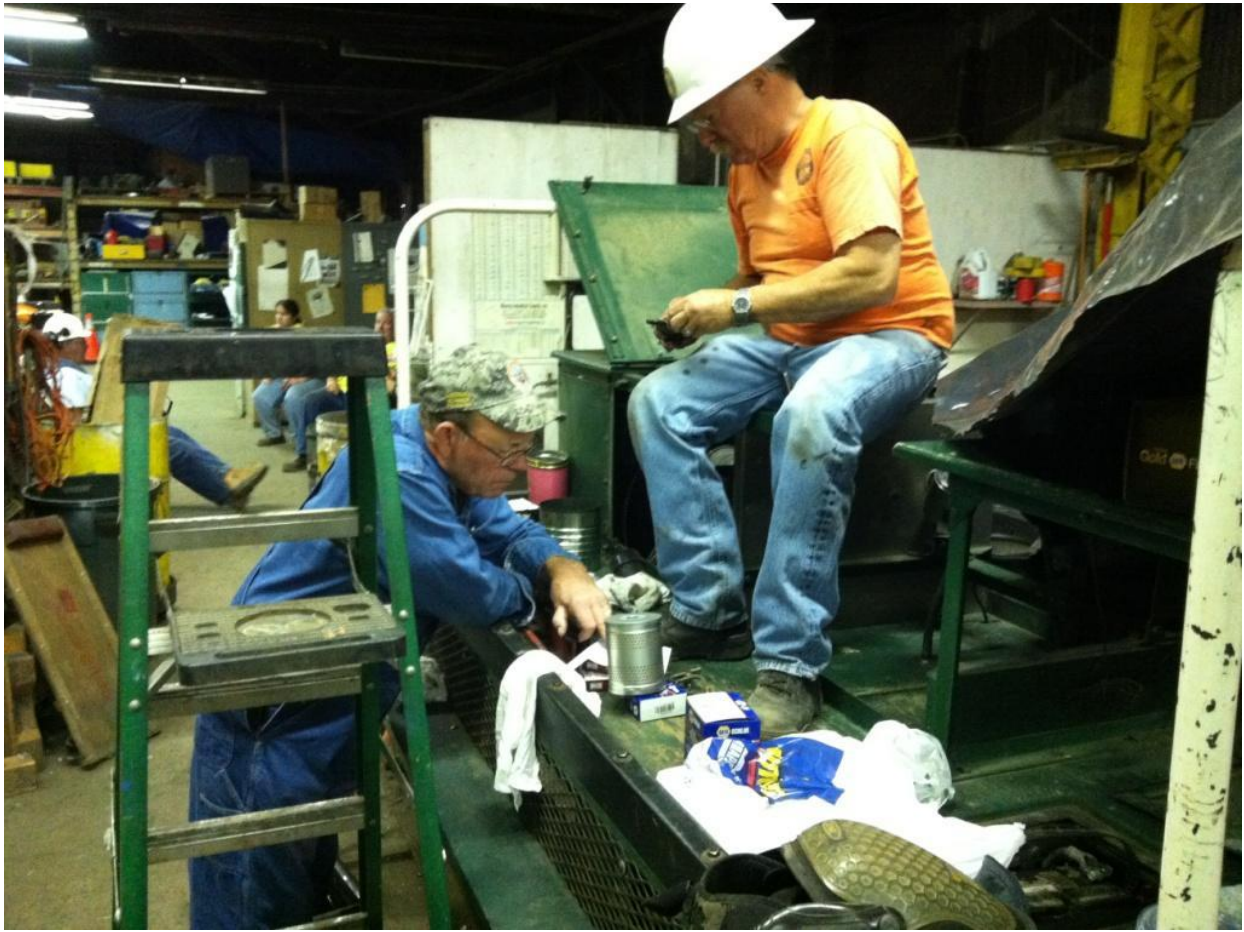
Cliff and Mike H. finish up work on the A-6 motorcar
