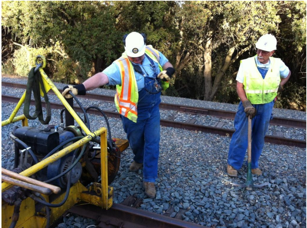
Chris pull-starts the section gang machine while Clem digs out the tie-ends
