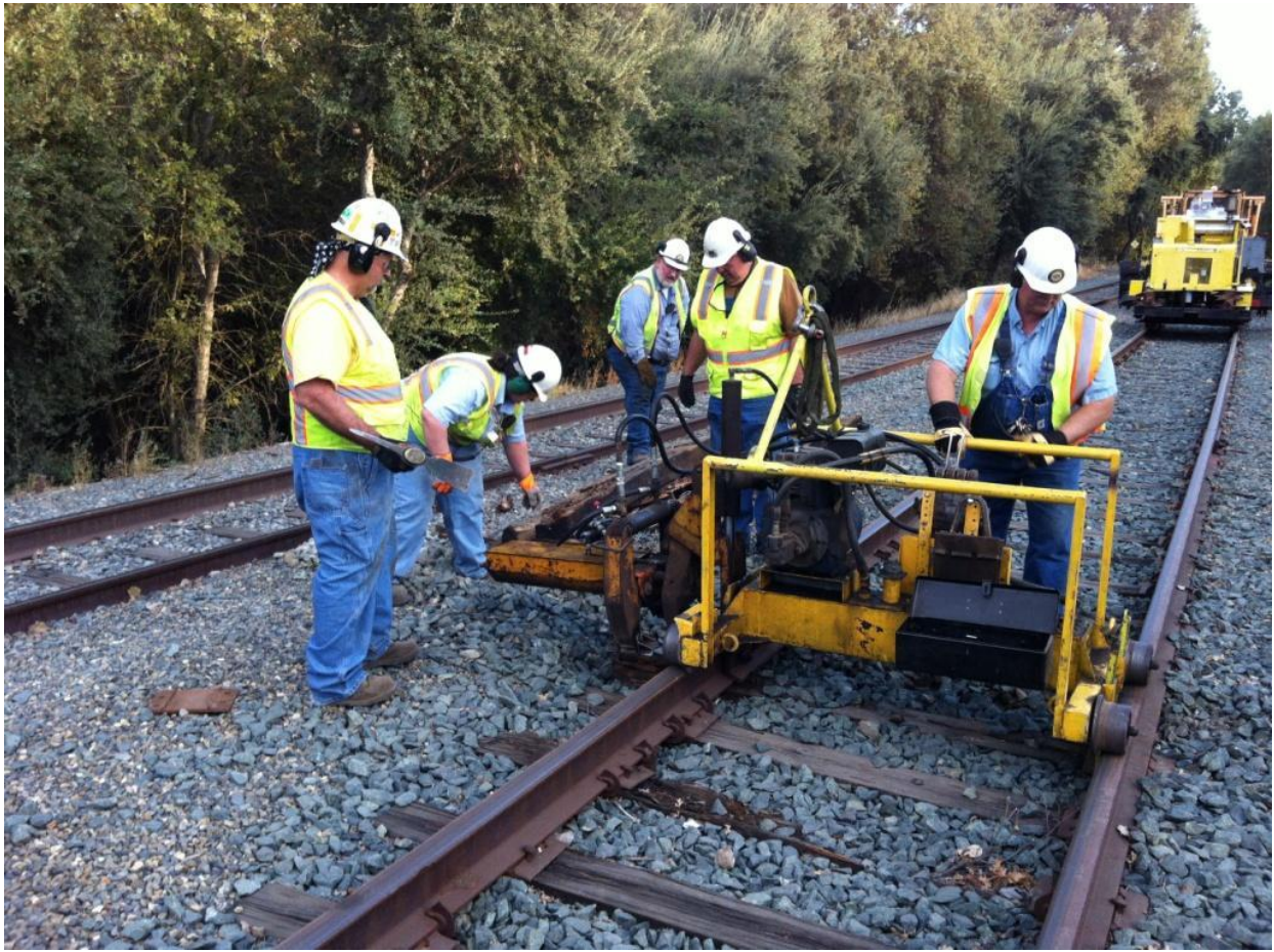
Mike F., Heather, Frank, Harry, and Chris pull our "demonstration" tie
