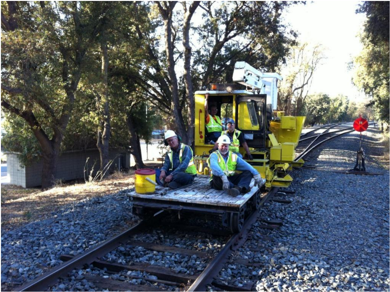
Steve, Mike M., Mike F., and engineer John back from dumping ties at Setzer
